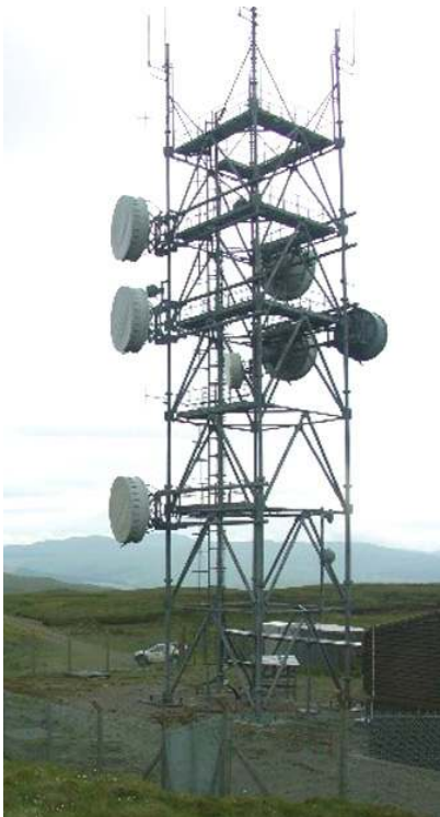
Figure 6a. Microwave repeater showing multiple co-located antennas. 3
